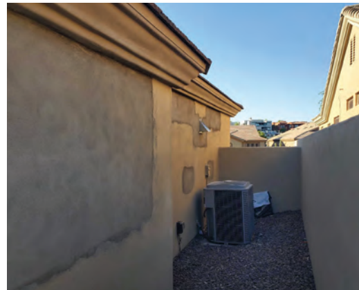
One of the best parts of this kitchen remodel was removing the small, decorative windows that distracted from the overall design. Filling them in allowed for a full wall of sleek slab-panel cabinetry, creating clean lines and a more cohesive, visually balanced kitchen.
