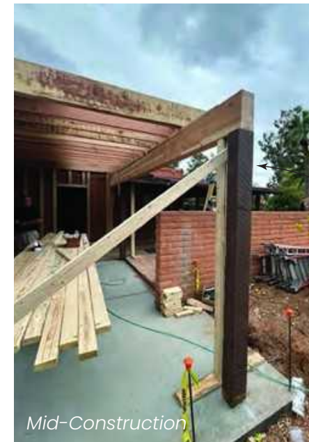
Re-purposed oak beams
